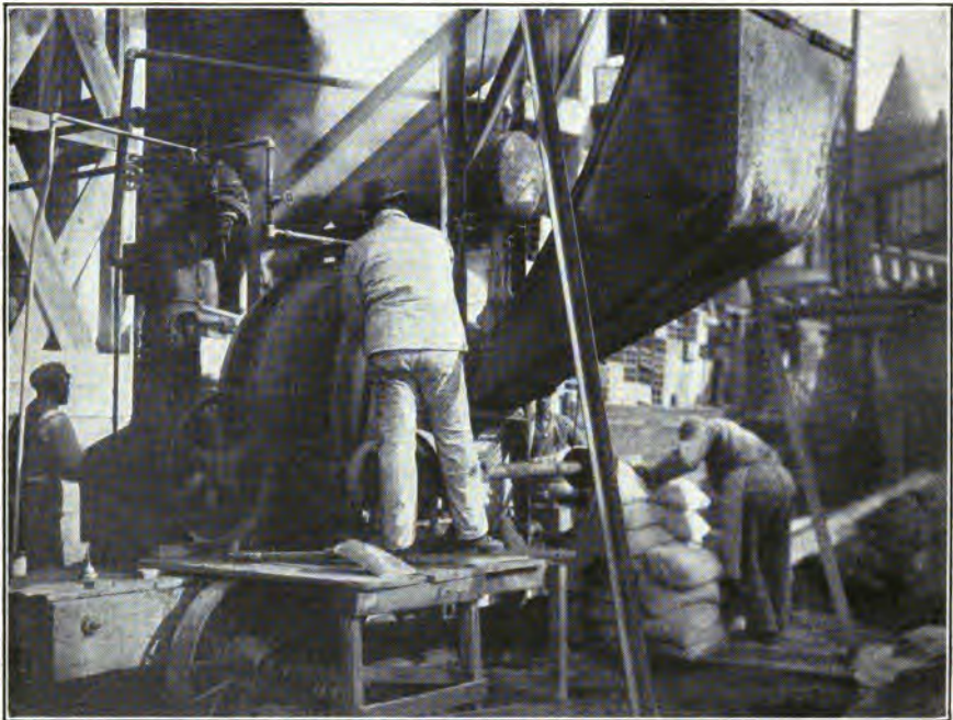
FIG. 1.—HEATED WATER BEING DISCHARGED DIRECTLY INTO MIXER.
